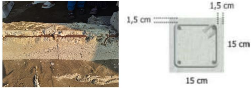
Figure 3. Thickness Blanket Concrete
