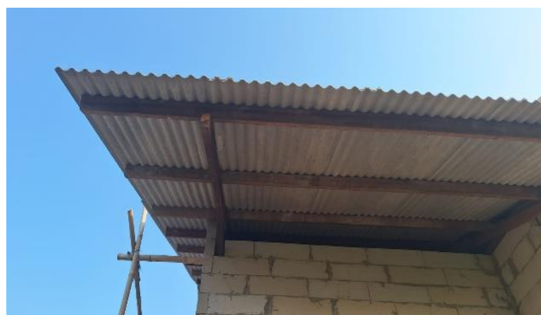
Figure 2. Usage Asbestos As Main Roof Covering
