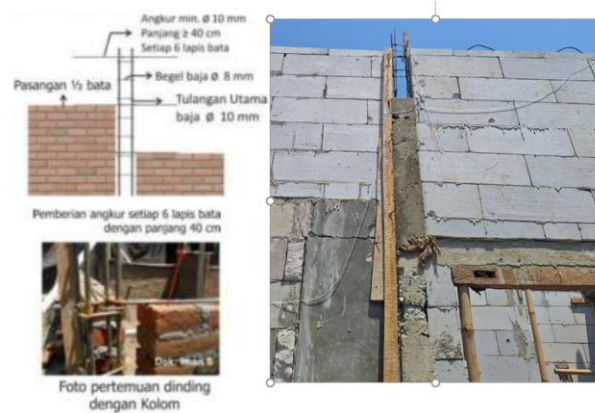
Figure 4. Anchor Reinforcement and Condition of Casting Results
